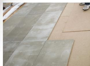
PANNELLI IN CEMENTO LEGNO PRESSATO IN LASTRE AD ELEVATA COMPATTEZZA, DENSITÀ E DUREZZA, RESISTENTI AL FUOCO, AGLI AGENTI ATMOSFERICI, CON OTTIME CARATTERISTICHE DI ISOLAMENTO TERMO-ACUSTICO
